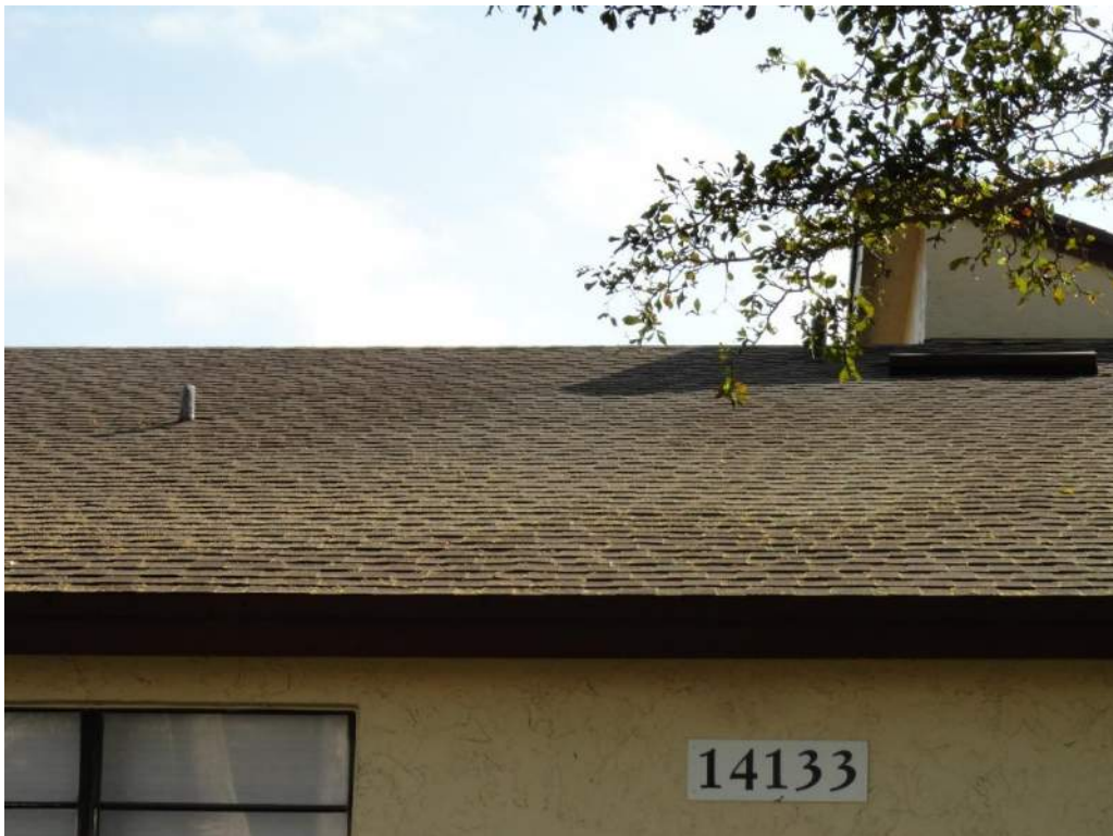
2. Roof Covering – Asphalt Shingles
