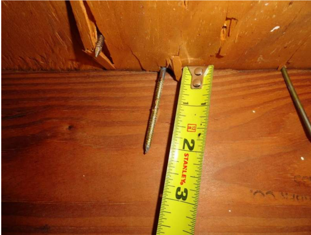
3. Roof Deck Attachment – 8d Nails
