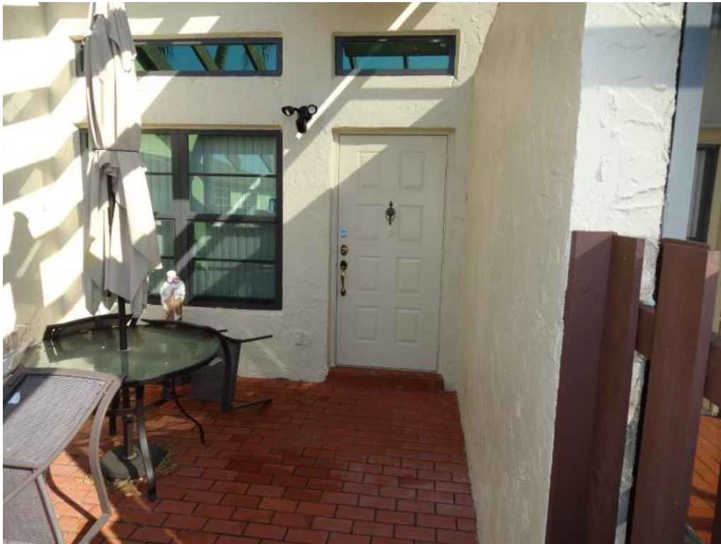
7. Opening Protection – Unprotected Unrated Unglazed Entry Door
