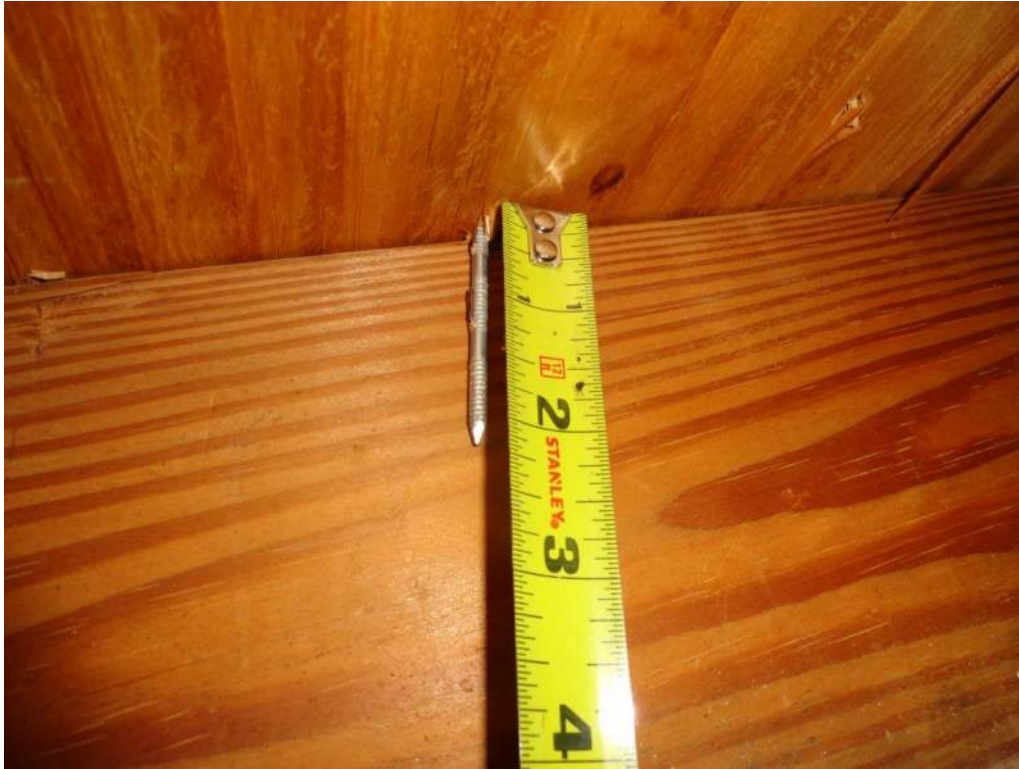
3. Roof Deck Attachment – 8d Nails
