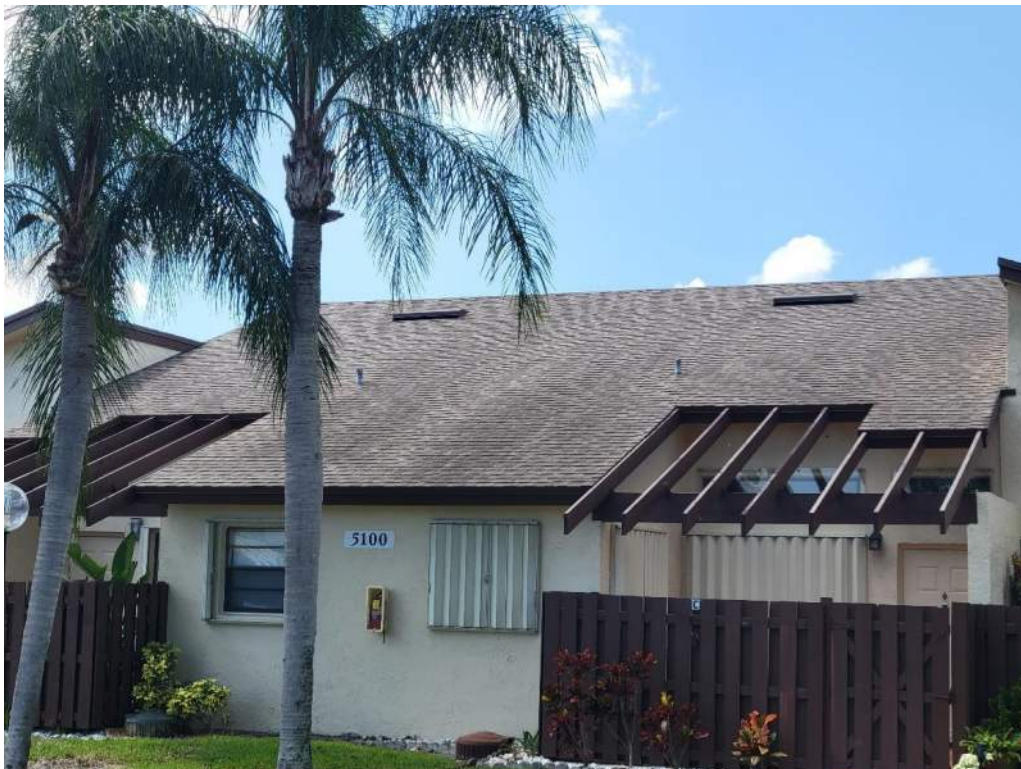
2. Roof Covering – Asphalt Shingles
