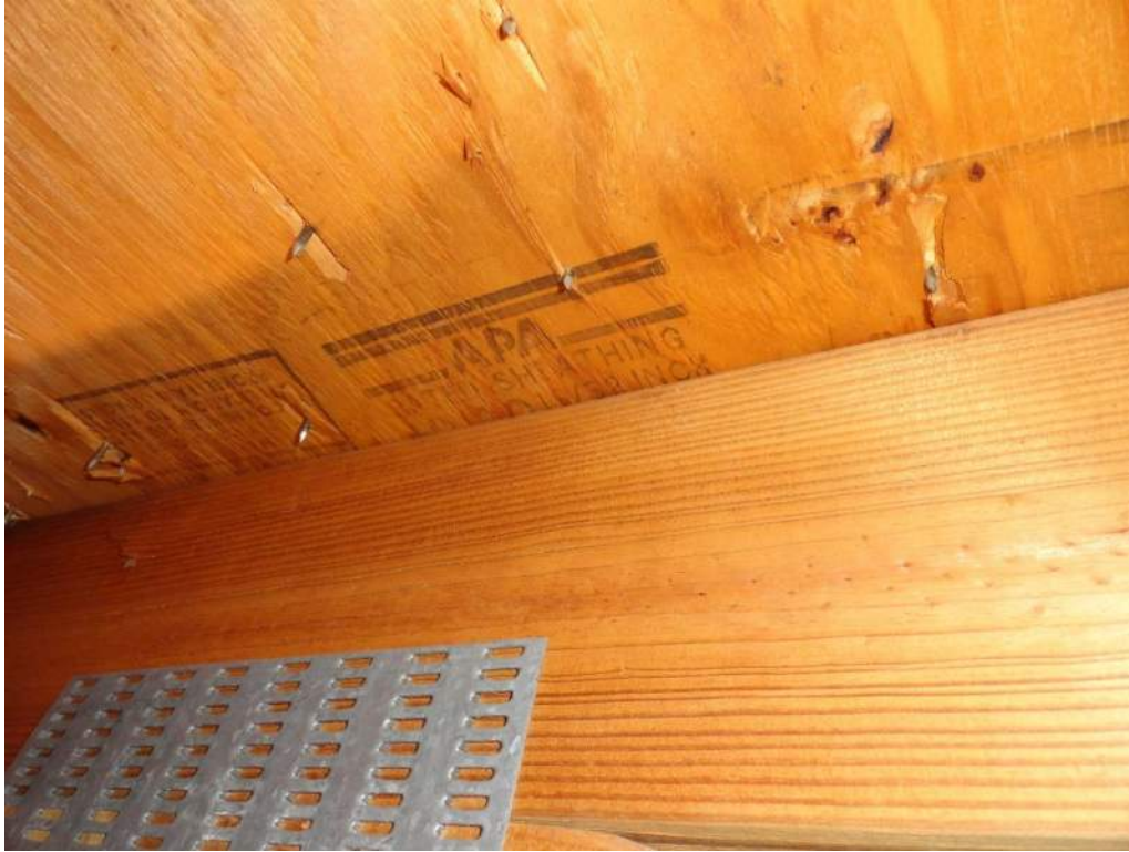
3. Roof Deck Attachment – 19/32" Plywood
