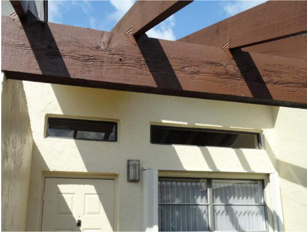
7. Opening Protection – Unrated Unprotected Windows
