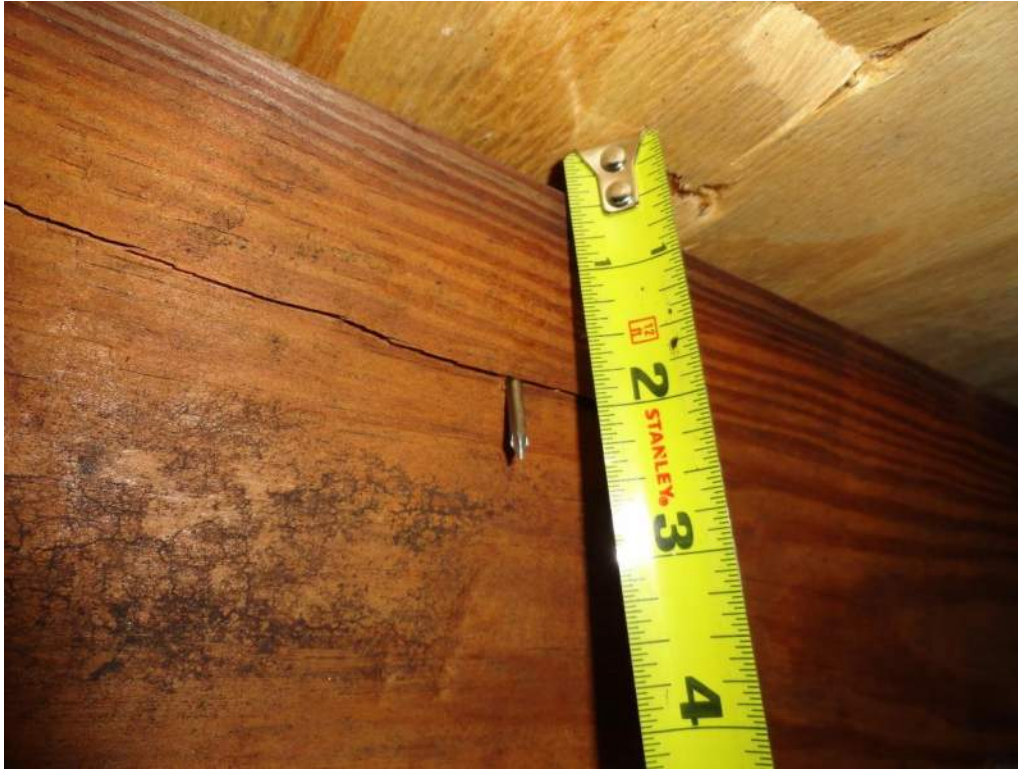
3. Roof Deck Attachment – 8d Nails
