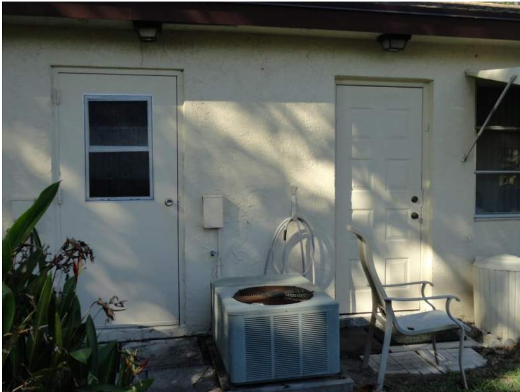
7. Opening Protection – Unprotected Unrated Unglazed Entry Door
