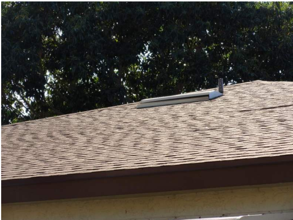
2. Roof Covering – Asphalt Shingles
