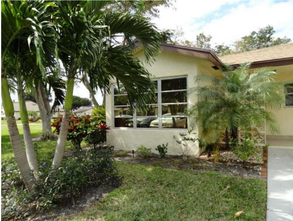
7. Opening Protection – Unrated Unprotected Windows
