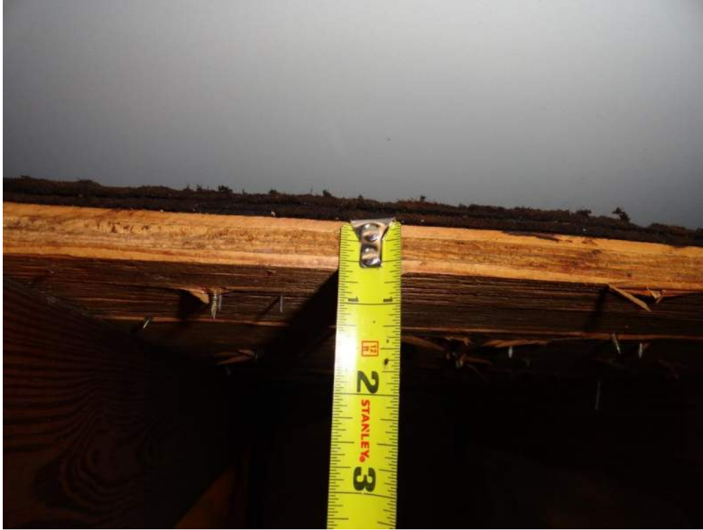
3. Roof Deck Attachment – 19/32" Plywood
