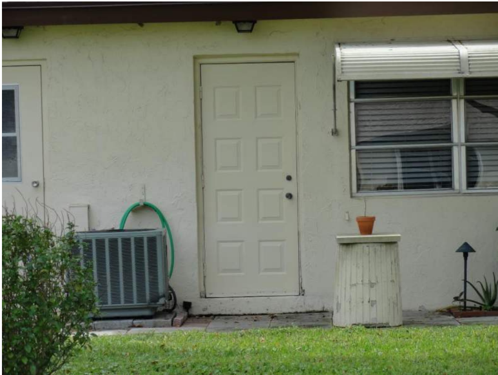
7. Opening Protection – Unprotected Unrated Unglazed Entry Door
