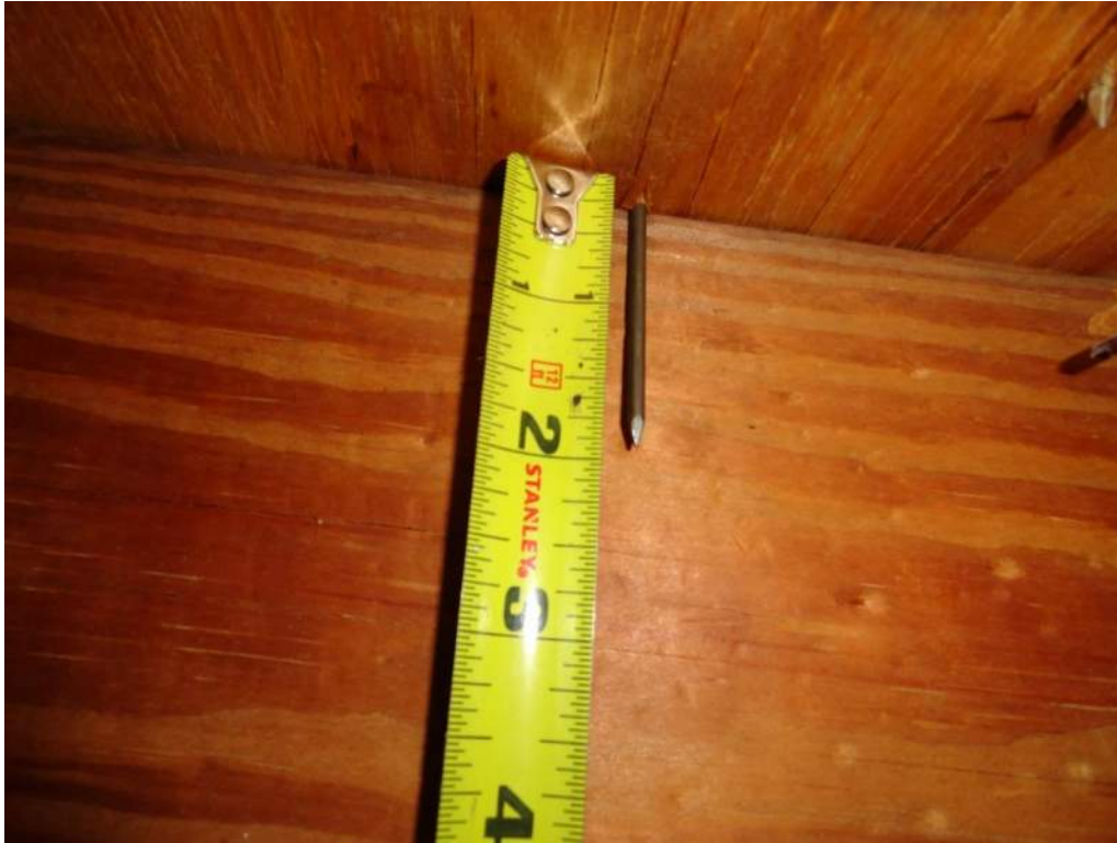
3. Roof Deck Attachment – 8d Nails
