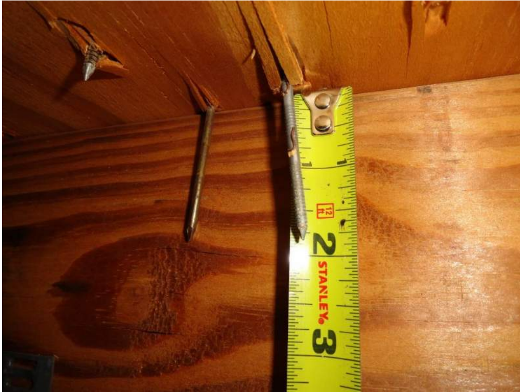
3. Roof Deck Attachment – 8d Nails
