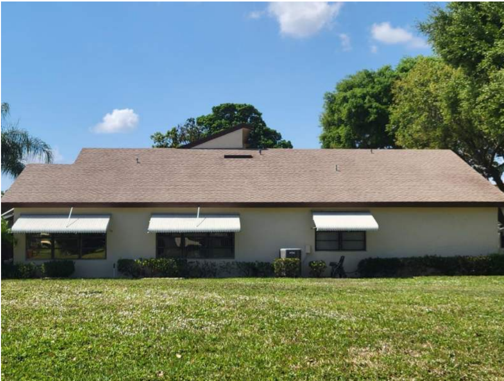
5. Roof Geometry – Right Elevation – Non-Hip
