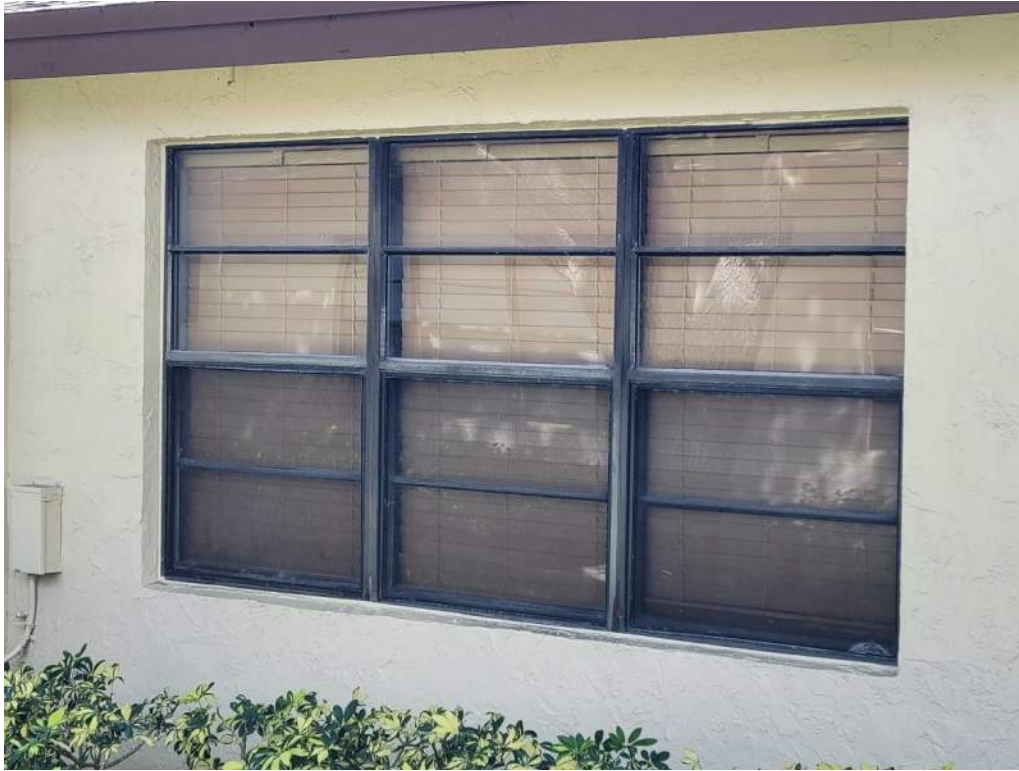
7. Opening Protection – Unrated Unprotected Windows
