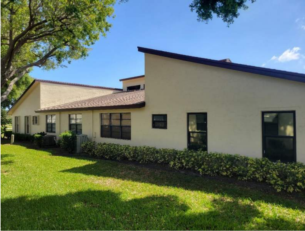
5. Roof Geometry – Rear Elevation – Non-Hip
