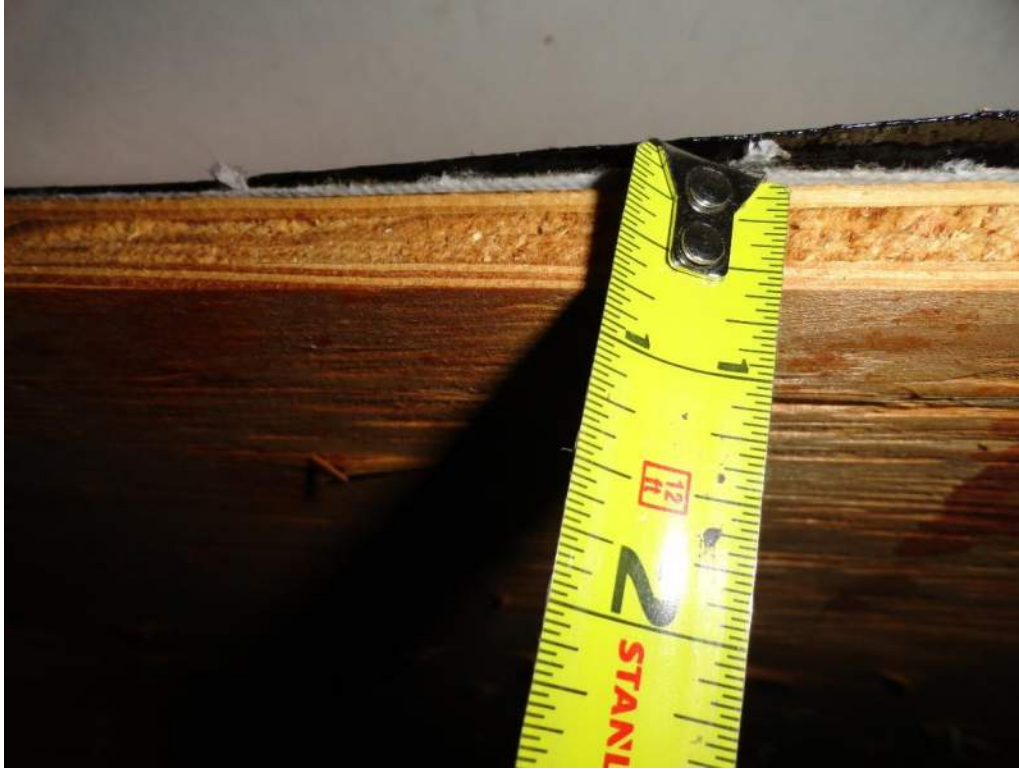
3. Roof Deck Attachment – 19/32" Plywood
