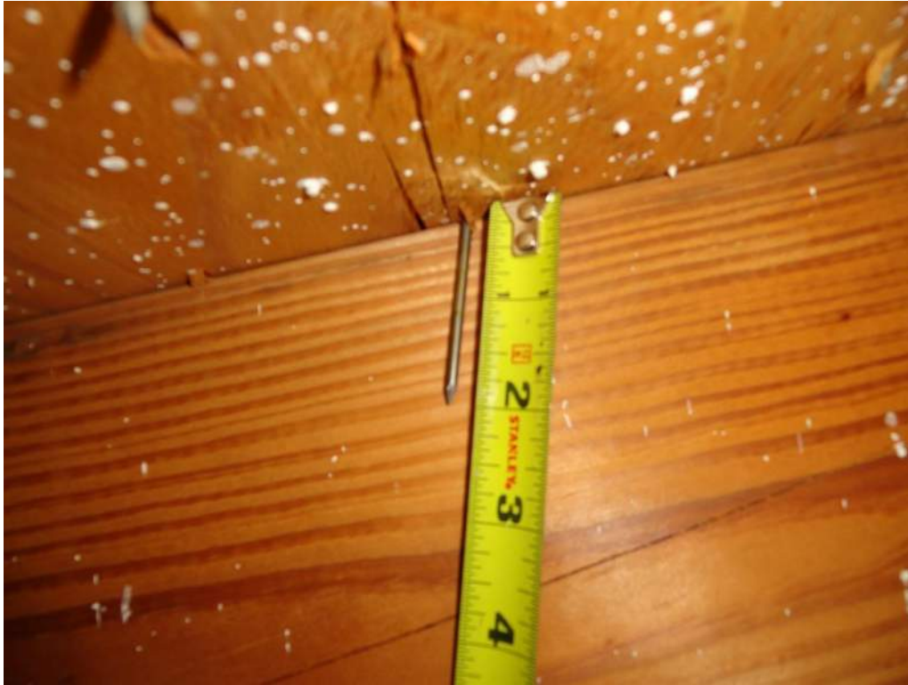
3. Roof Deck Attachment – 8d Nails
