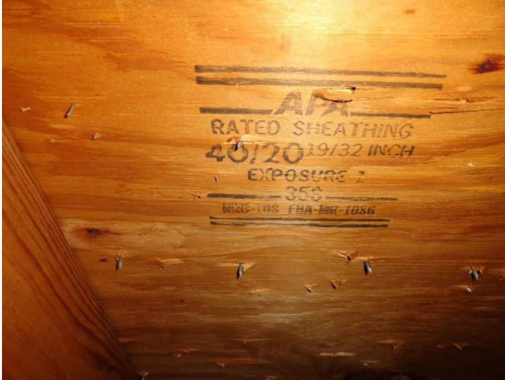
3. Roof Deck Attachment – 19/32" Plywood
