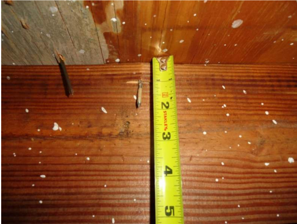
3. Roof Deck Attachment – 8d Nails
