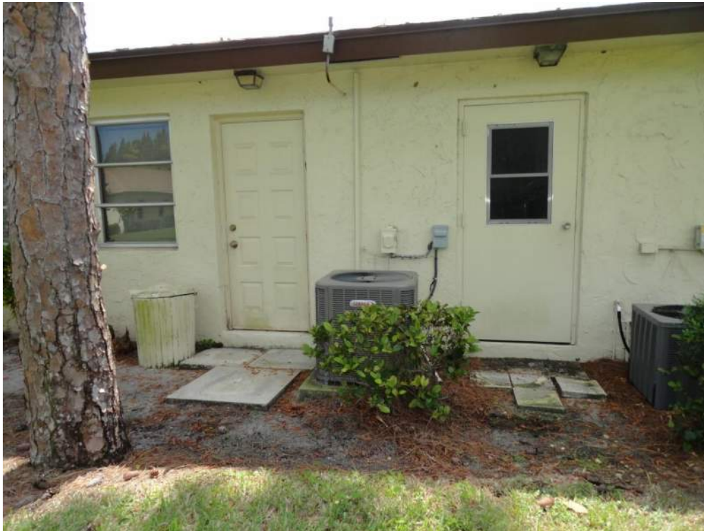
7. Opening Protection – Unprotected Unrated Unglazed Entry Door
