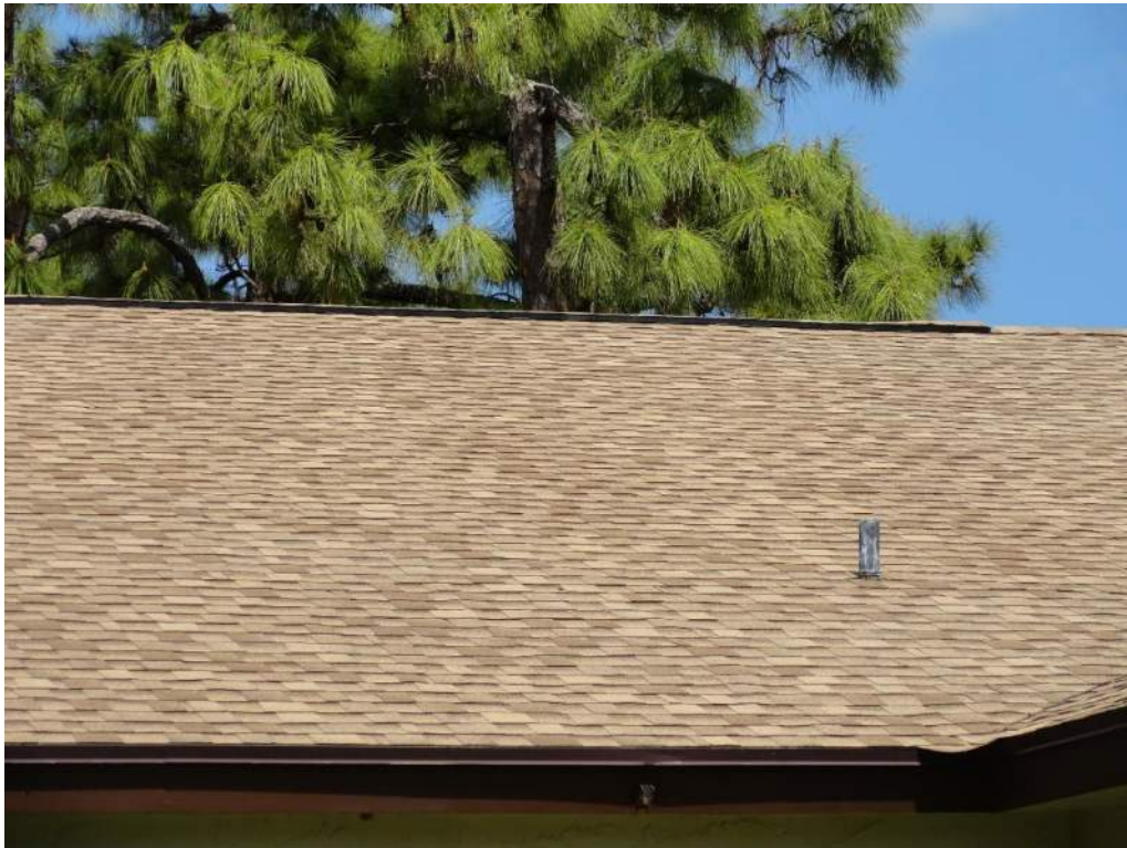
2. Roof Covering – Asphalt Shingles
