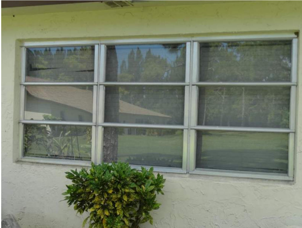
7. Opening Protection – Unrated Unprotected Windows
