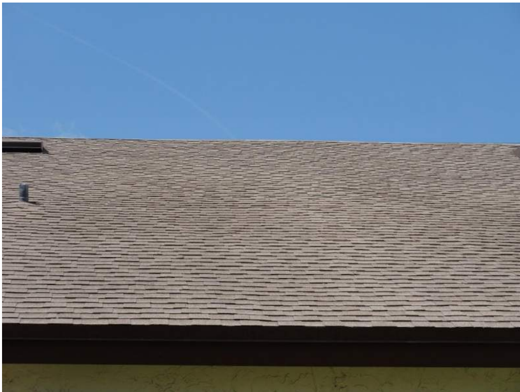
2. Roof Covering – Asphalt Shingles
