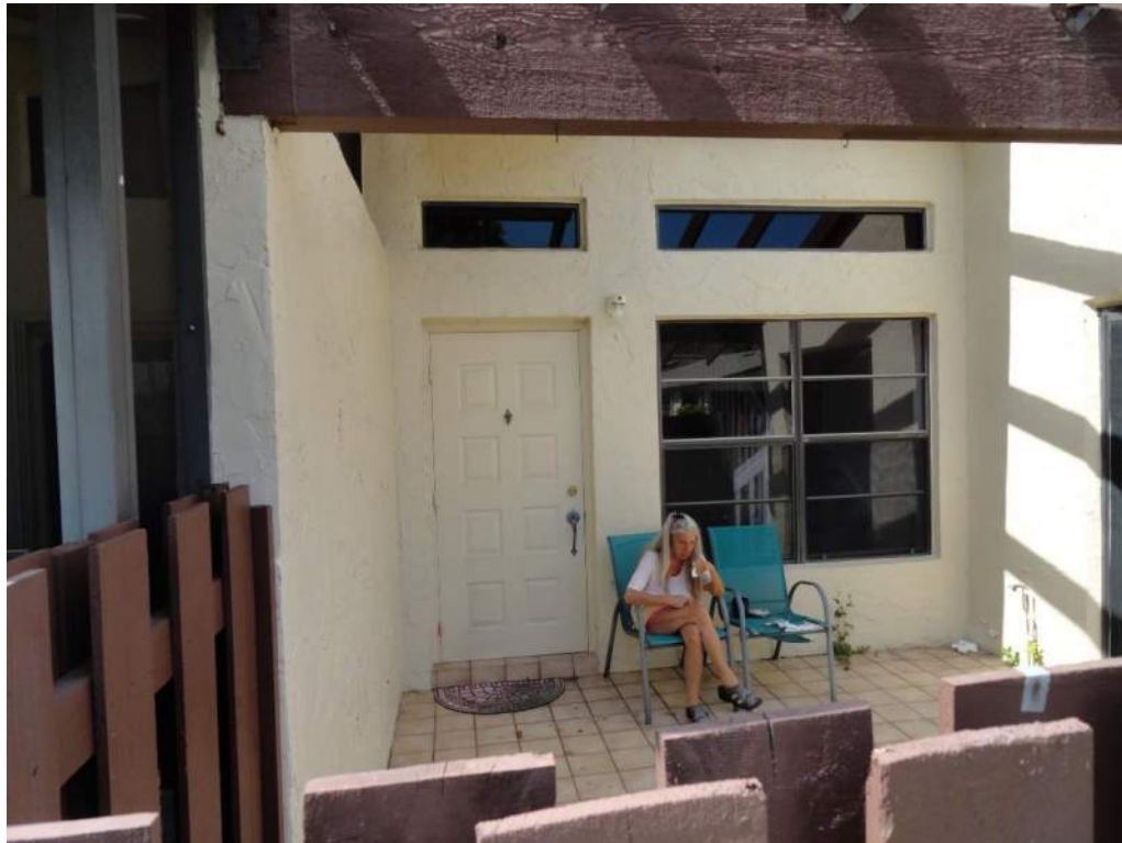
7. Opening Protection – Unprotected Unrated Unglazed Entry Door
