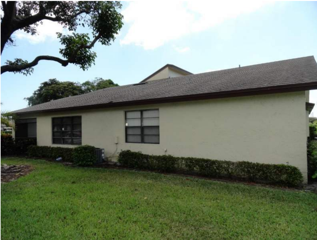
5. Roof Geometry – Right Elevation – Non-Hip
