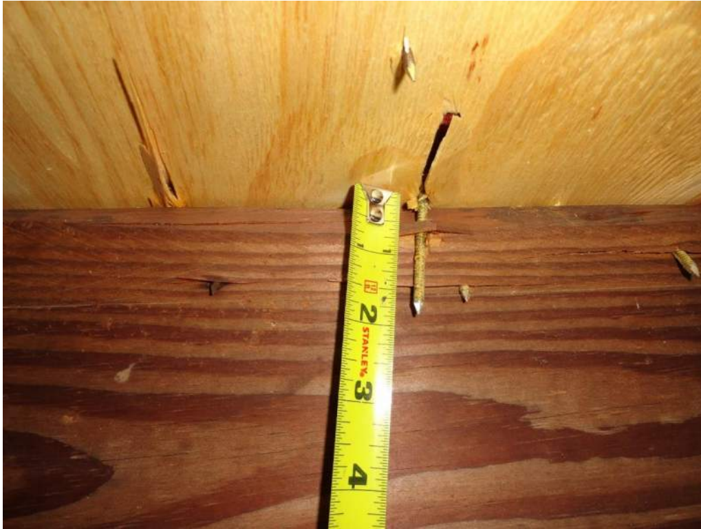
3. Roof Deck Attachment – 8d Nails
