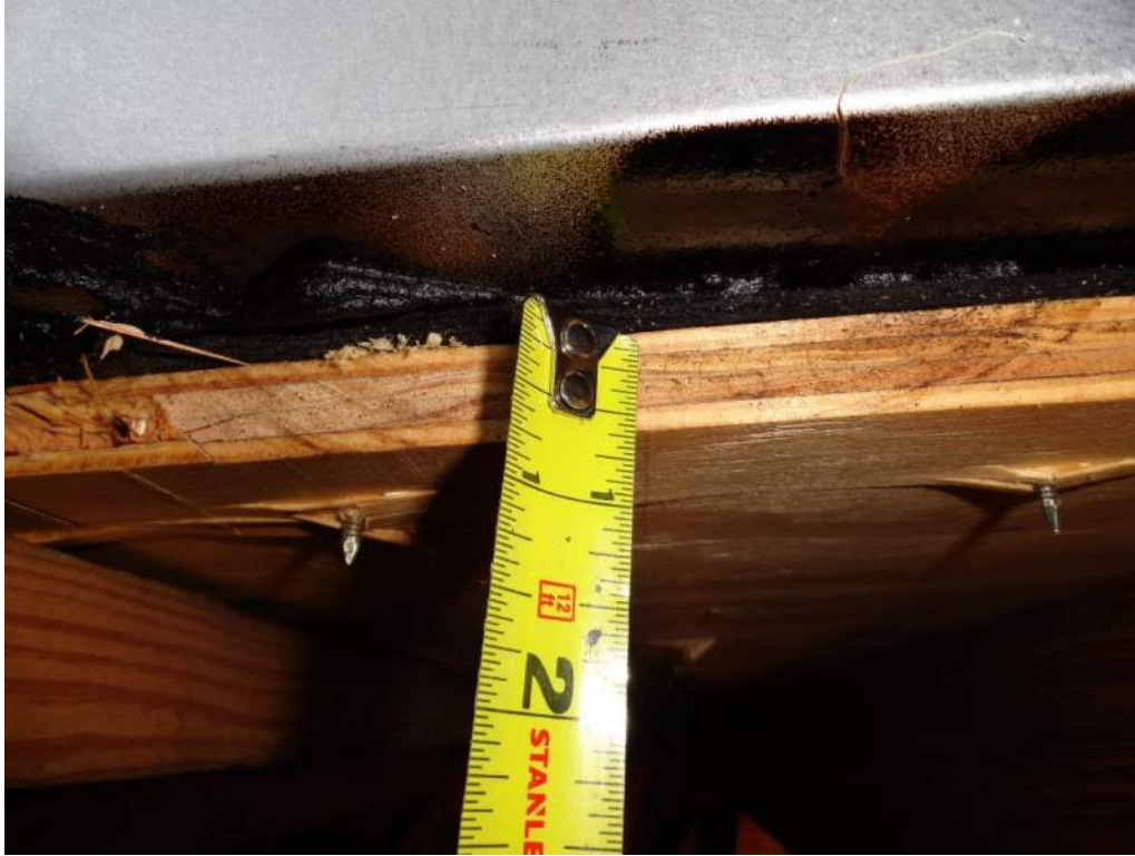
3. Roof Deck Attachment – 5/8" Plywood
