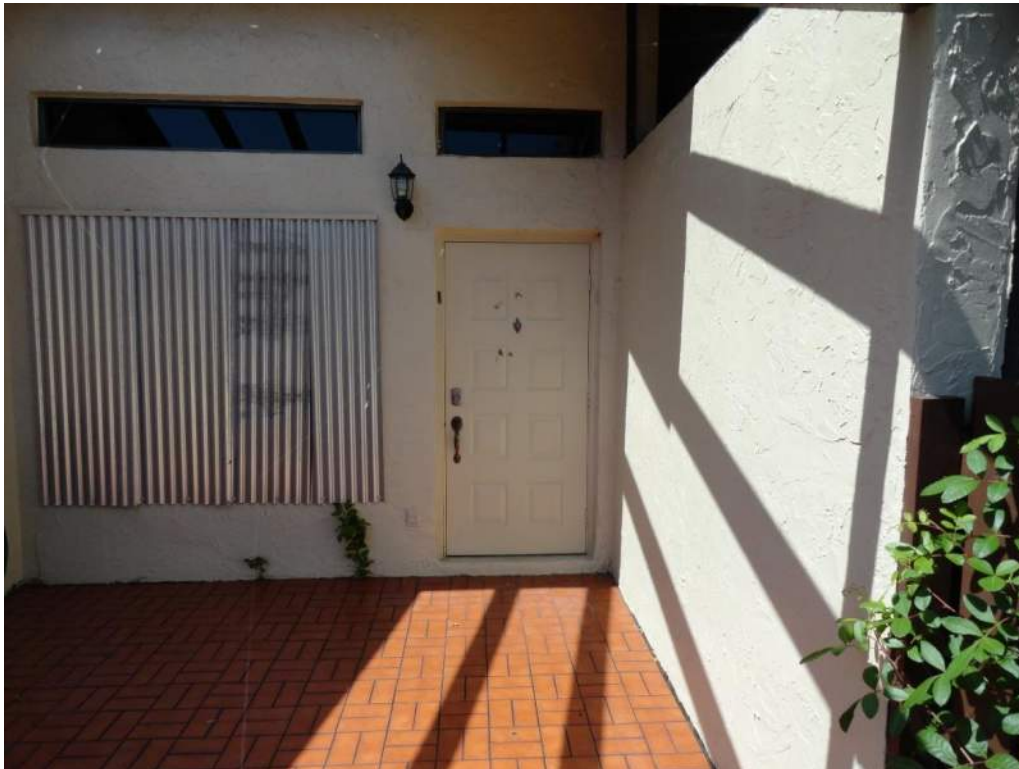
7. Opening Protection – Unprotected Unrated Unglazed Entry Door
