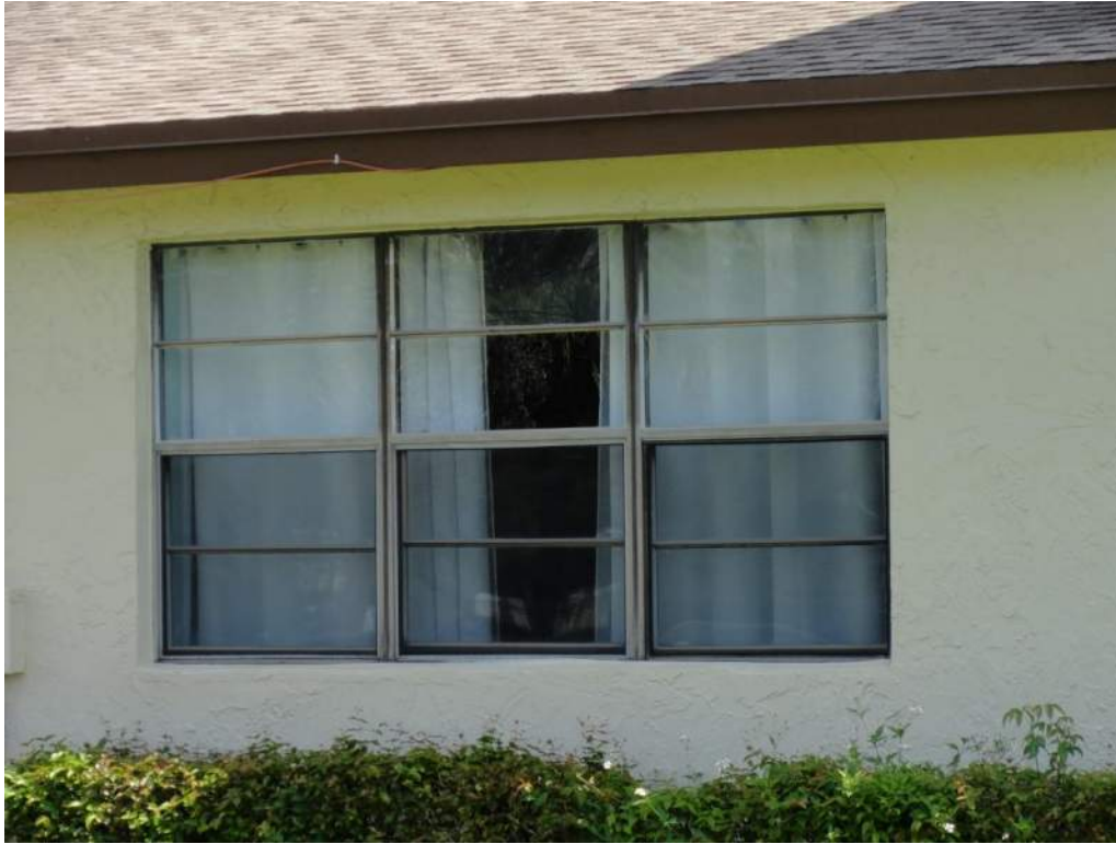
7. Opening Protection – Unprotected Unrated Windows
