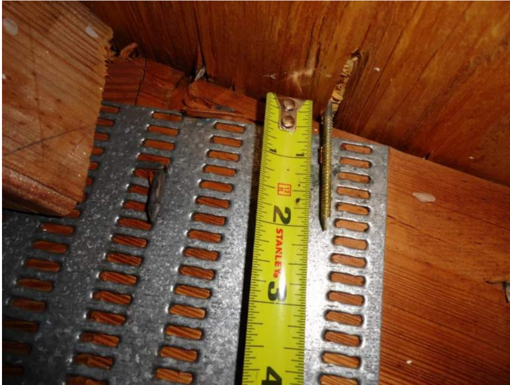
3. Roof Deck Attachment – 8d Nails
