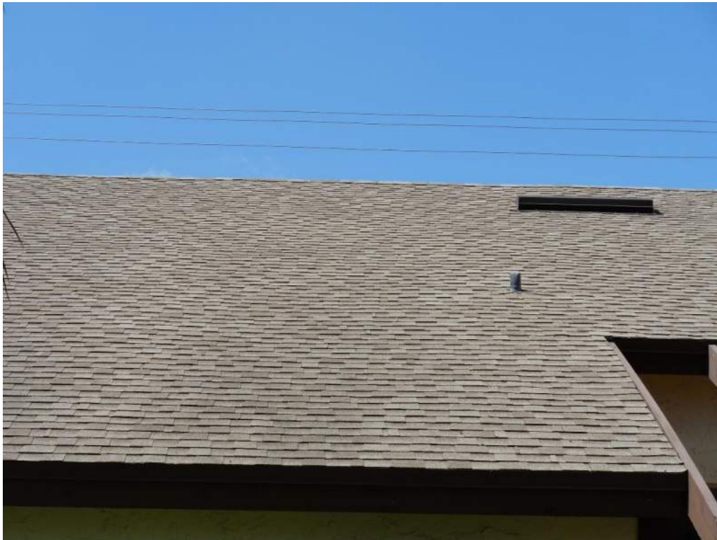
2. Roof Covering – Asphalt Shingles
