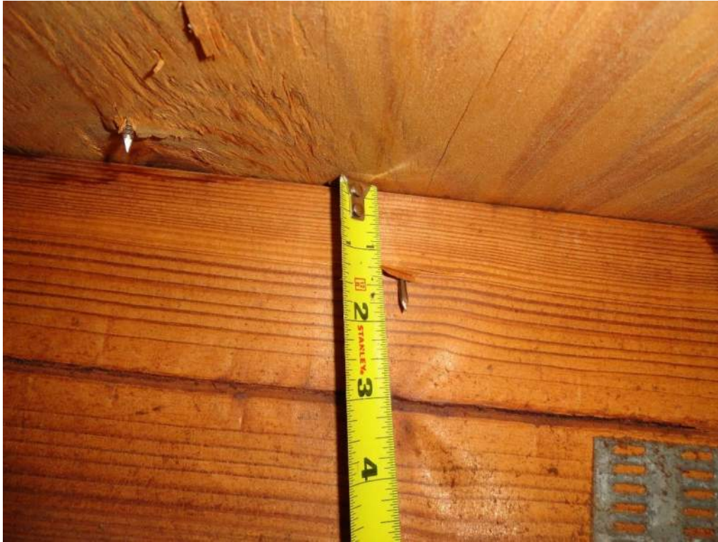
3. Roof Deck Attachment – 8d Nails
