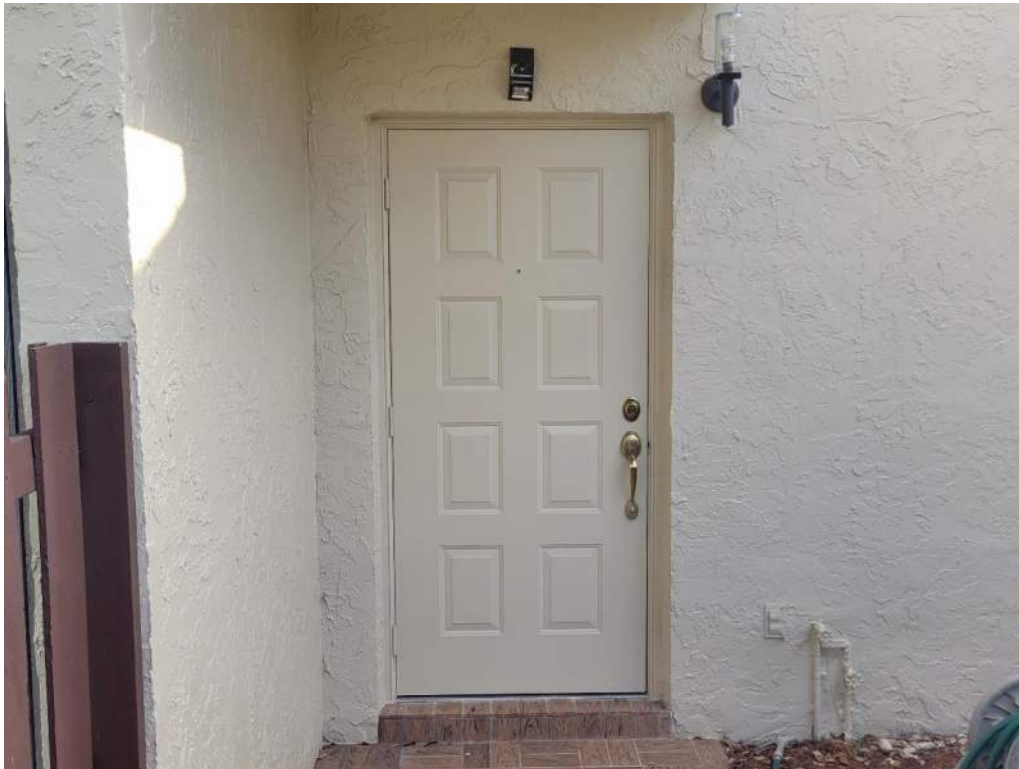
7. Opening Protection – Unprotected Unrated Unglazed Entry Door
