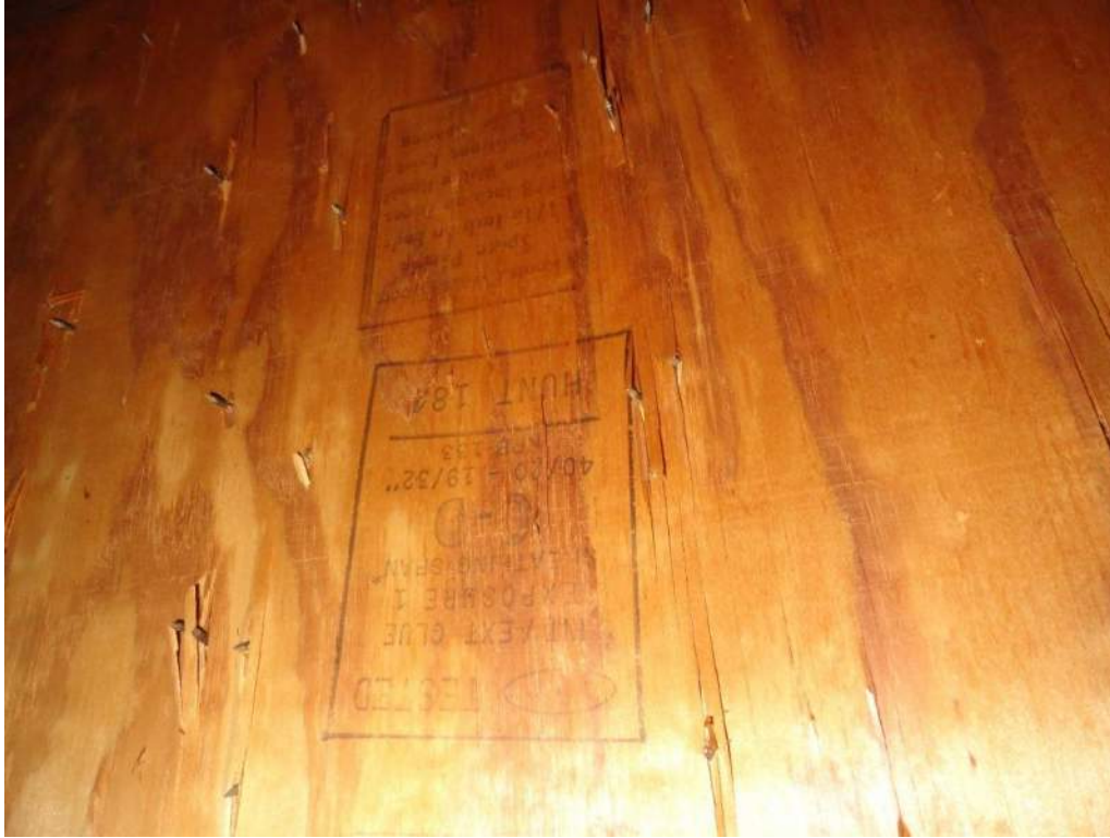
3. Roof Deck Attachment – 19/32" Plywood
