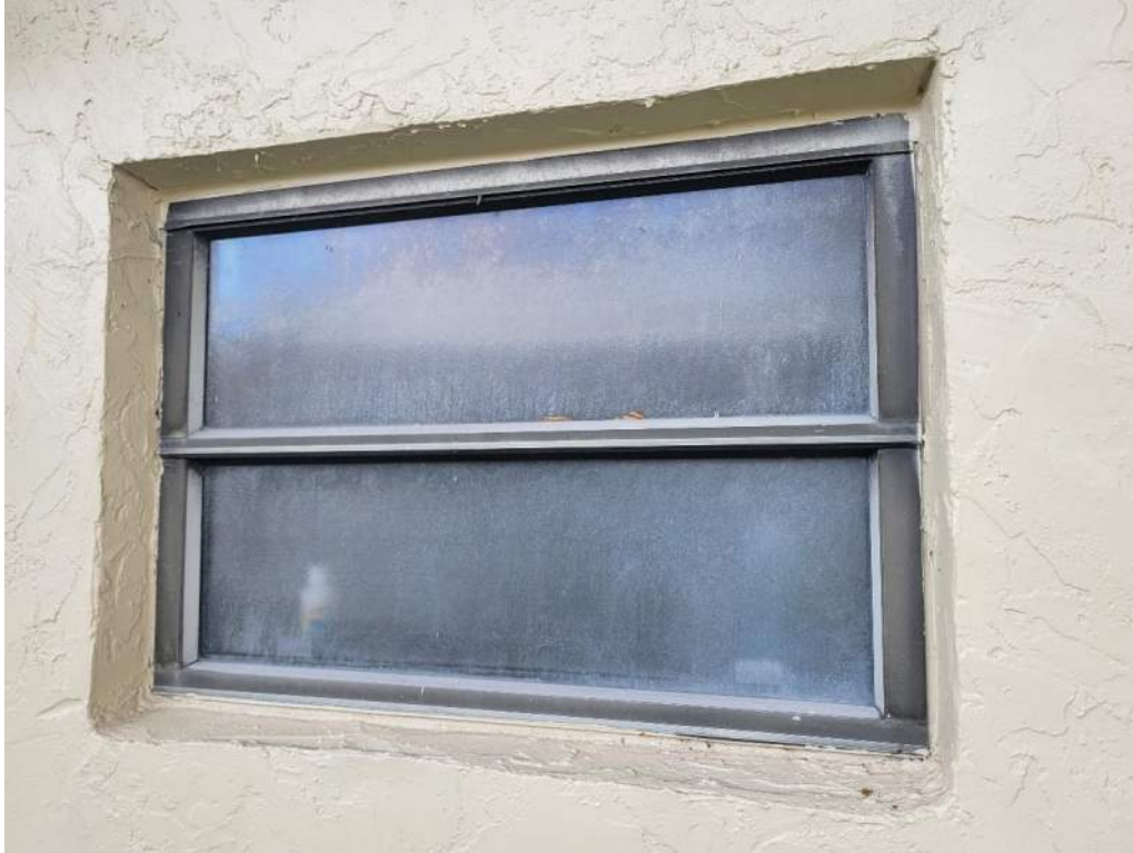
7. Opening Protection – Unrated Unprotected Windows
