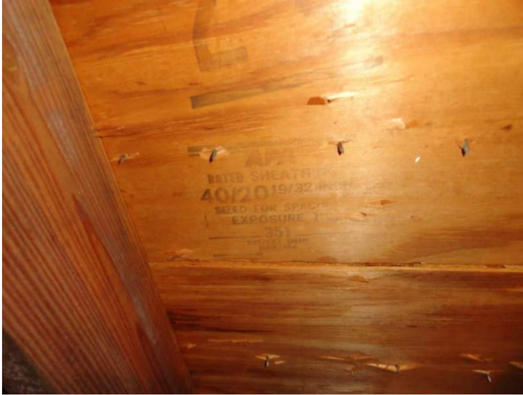
3. Roof Deck Attachment – 19/32" Plywood
