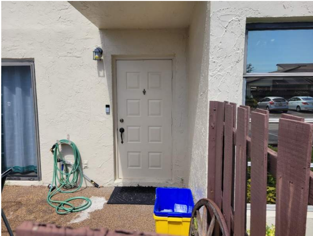
7. Opening Protection – Unprotected Unrated Unglazed Entry Door
