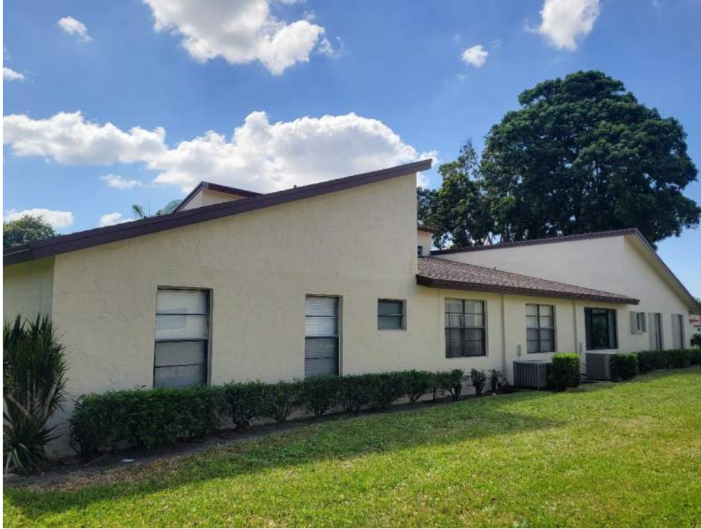
5. Roof Geometry – Rear Elevation – Non-Hip
