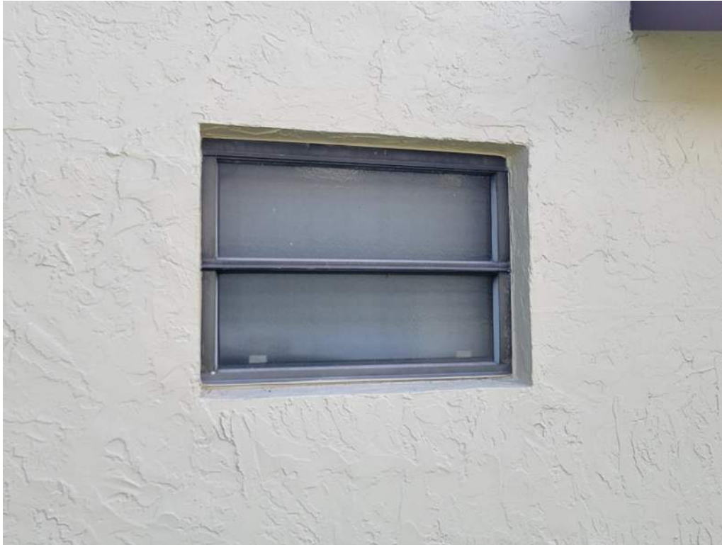
7. Opening Protection – Unrated Unprotected Windows
