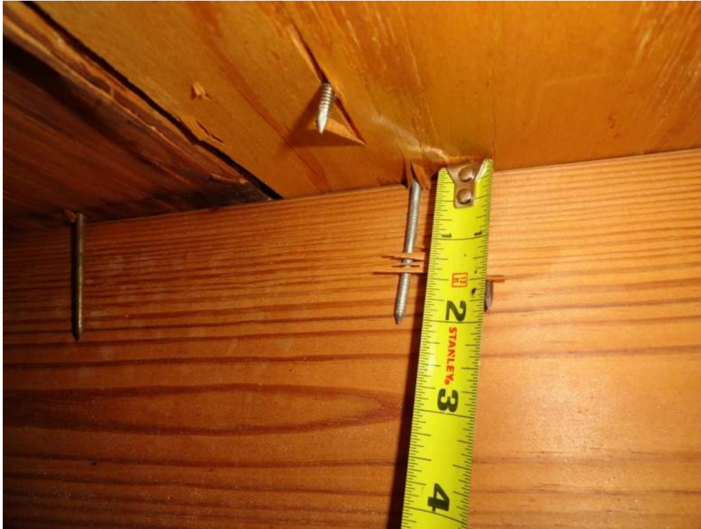
3. Roof Deck Attachment – 8d Nails
