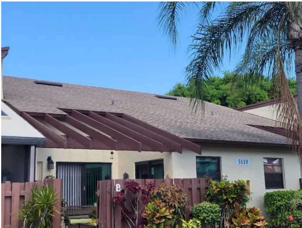
2. Roof Covering – Asphalt Shingles
