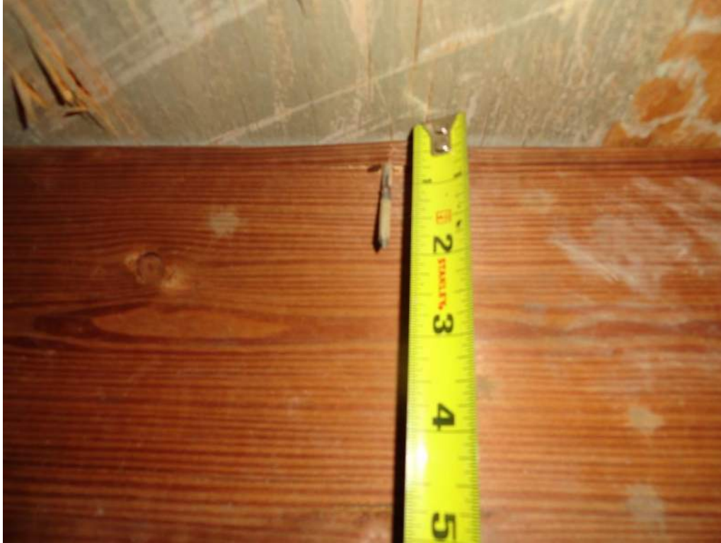
3. Roof Deck Attachment – 8d Nails
