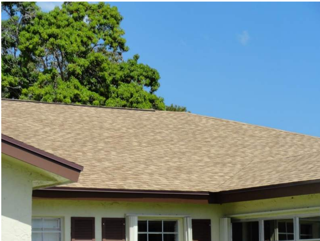
2. Roof Covering – Asphalt Shingles
