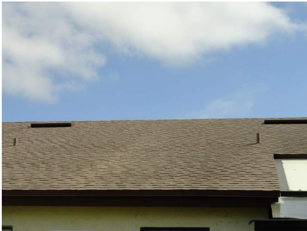
2. Roof Covering – Asphalt Shingles
