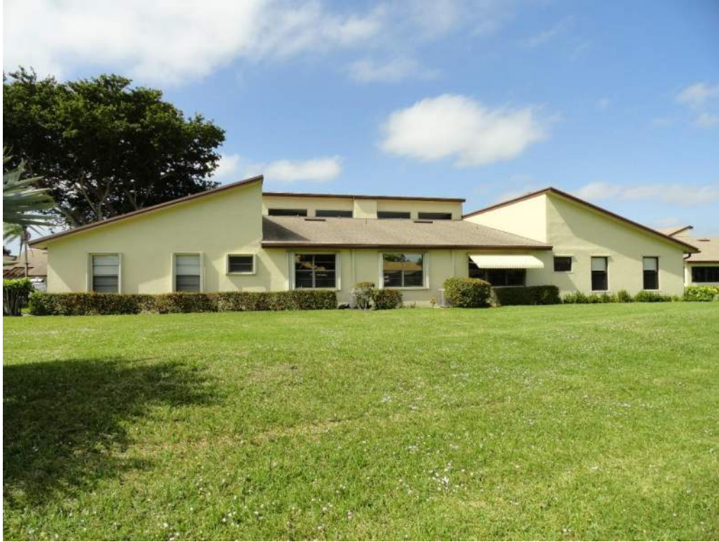
5. Roof Geometry – Rear Elevation – Non-Hip
