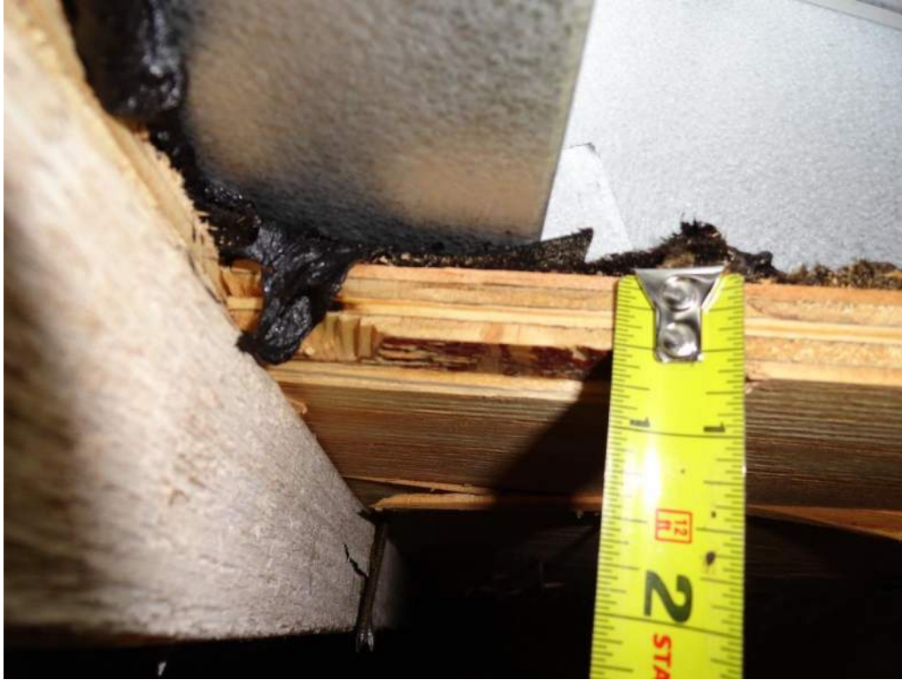
3. Roof Deck Attachment – 19/32" Plywood
