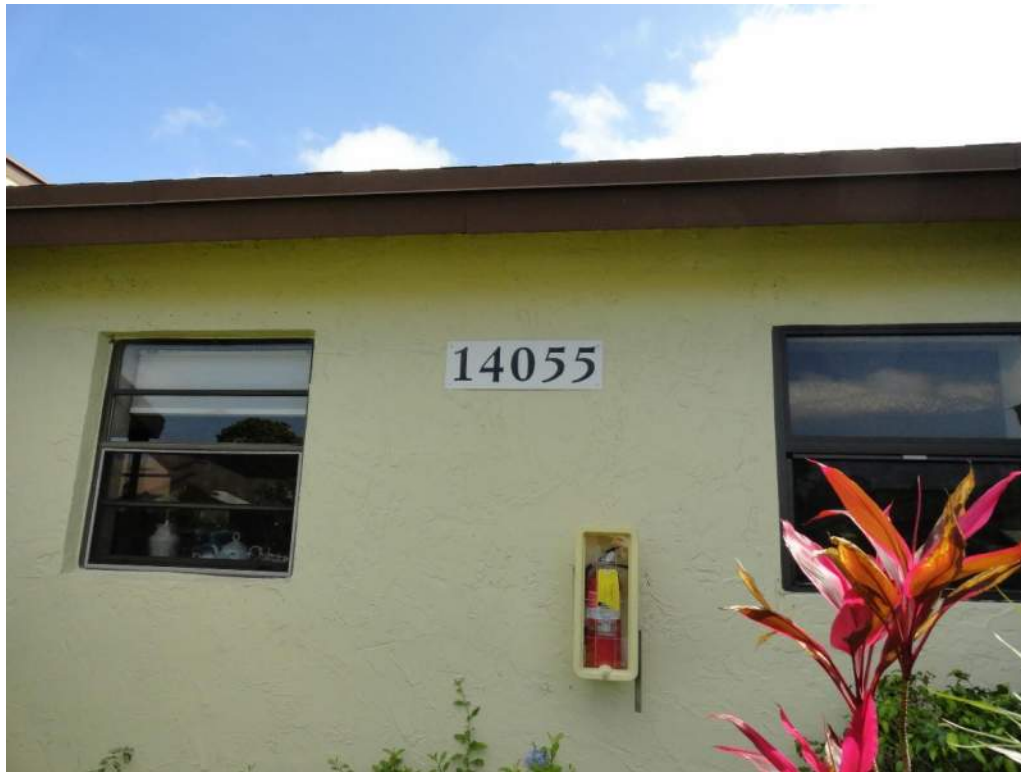
7. Opening Protection – Unrated Unprotected Windows
