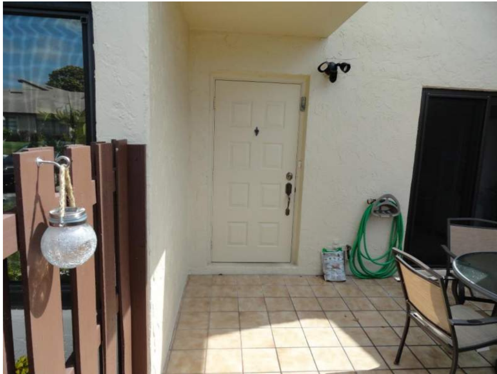
7. Opening Protection – Unprotected Unrated Unglazed Entry Door
