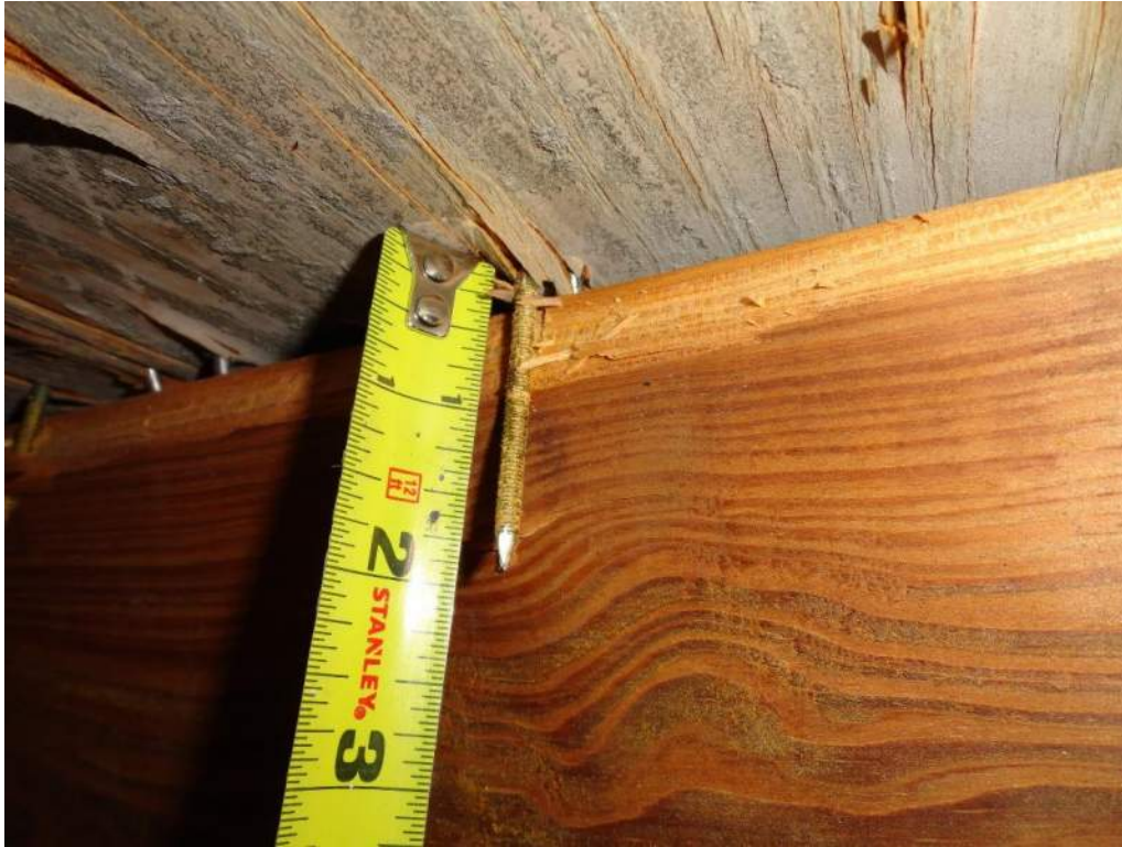
3. Roof Deck Attachment – 8d Nails
